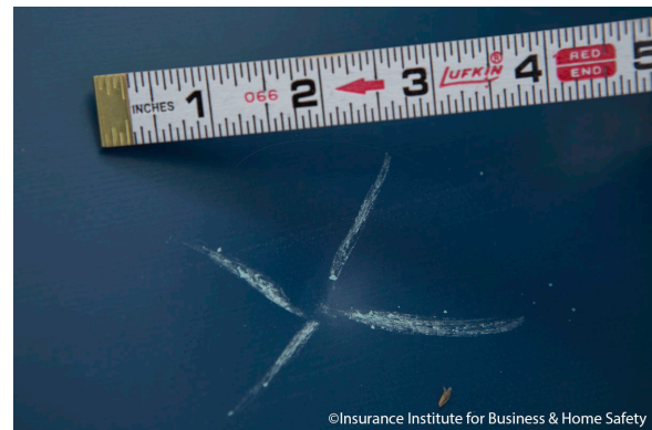
Although the damage to the test specimen's metal roof shown above is clearly visible, it was only cosmetic in nature.
